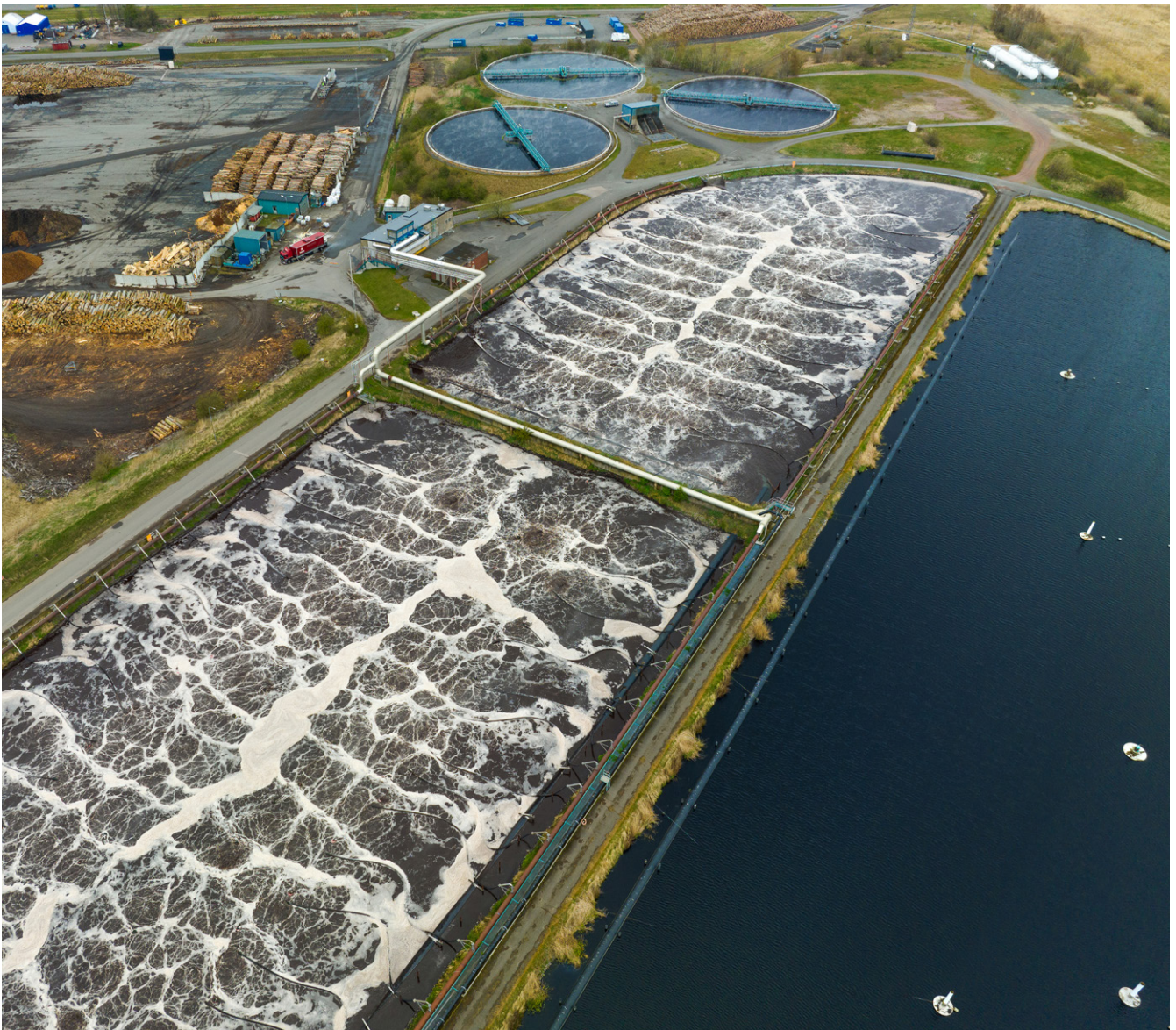
The activated sludge plant for biological treatment of wastewater.
