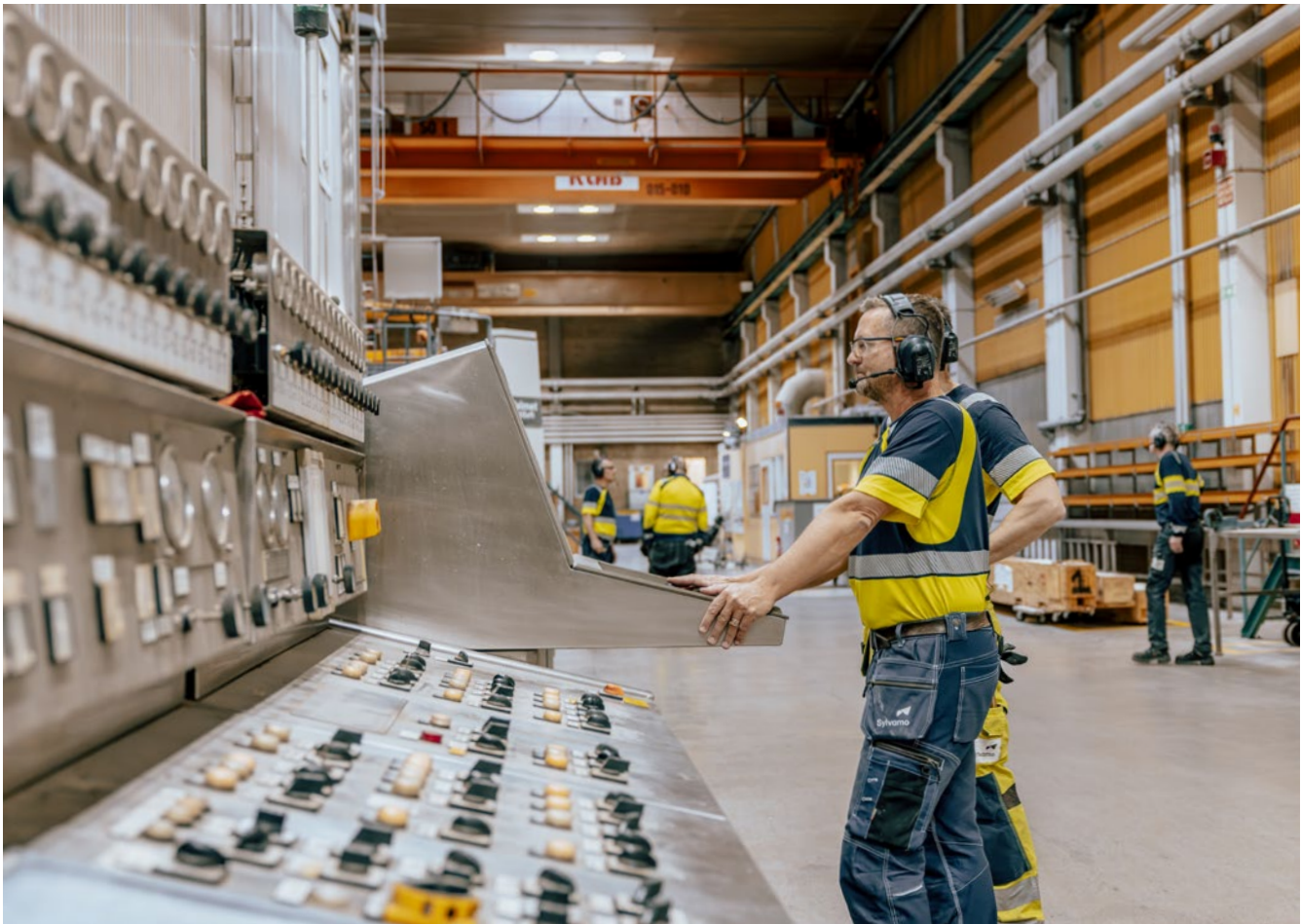
The control panel PM1
