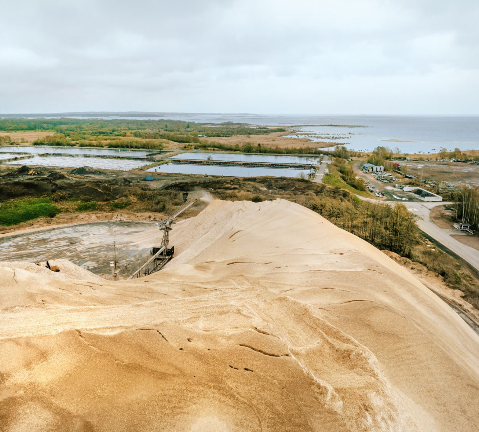
The Chip pile with the activated sludge plant in the background.
